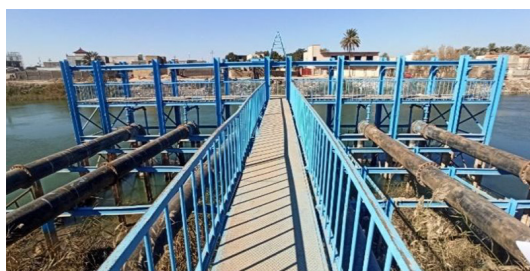
(a) Water collect unit.
