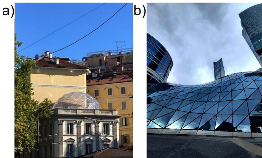
Figure 1. Example of lightweight structures: a) geodesic dome in a residential house in Milan (Italy), b) roof of a shopping mall in Warsaw (Poland)
