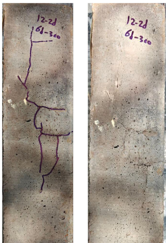
Figure 9. Cracks after exposing to 300 °C
