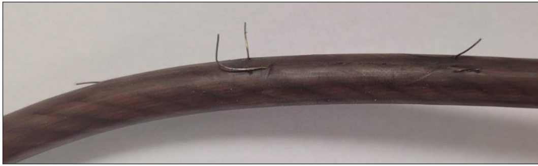
Figure 8. Damage to the wires of the CTP rope
