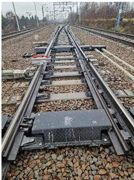
Figure 10. Tested switch: a) measurement of the curved switch rail, b) measurement locations
