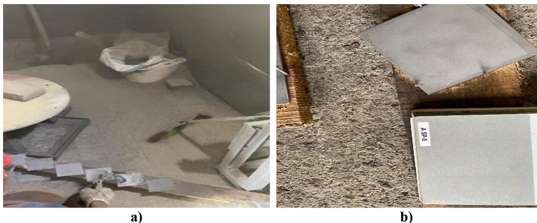
Figure 2. Sandblasting (a) and surface cleaning check (b)
