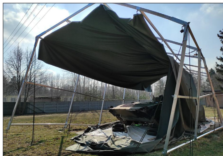
Figure 10. Destruction of NUPWU I (former model) as a result of hurricane Eunice during February 17–18, 2022, with wind speeds reaching 100÷120 km/h
