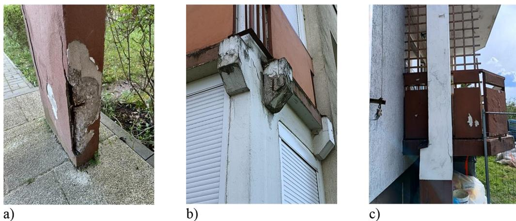
**Figure 1.** Damage images in structural elements of large-panel blocks: a) column at the entrance to the building, b) reinforced concrete bracket at the loggias, and c) column supporting the balcony
