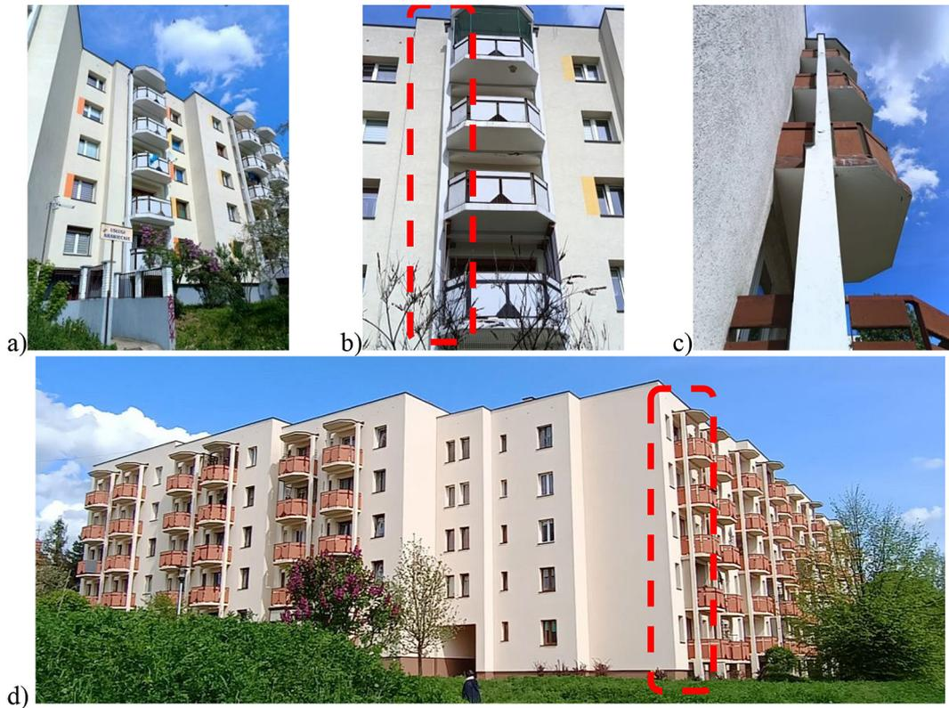
**Figure 5.** Flaccid columns supporting balconies in a buildings erected in large panel system
